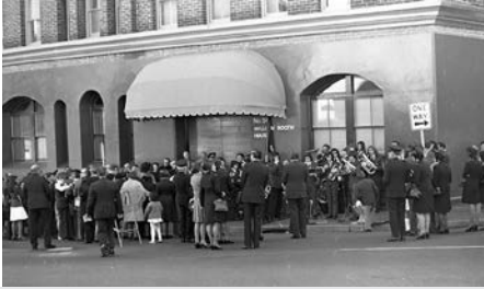
The opening of the William Booth House building in Sydney 100 years ago.
